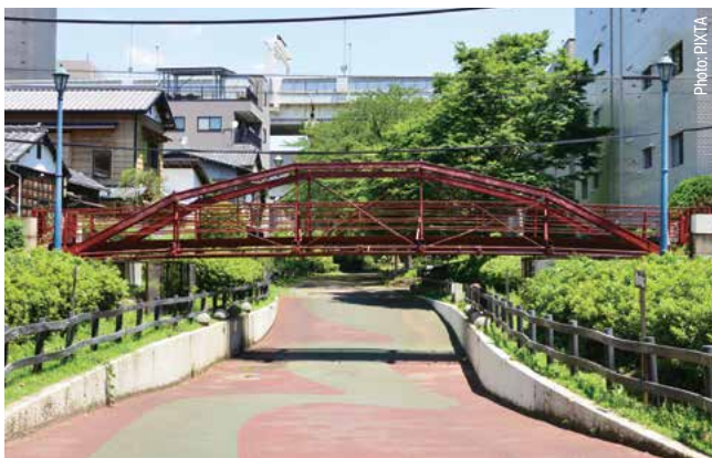
The Hachiman Bridge built in 1878 (Koto City, Tokyo)
