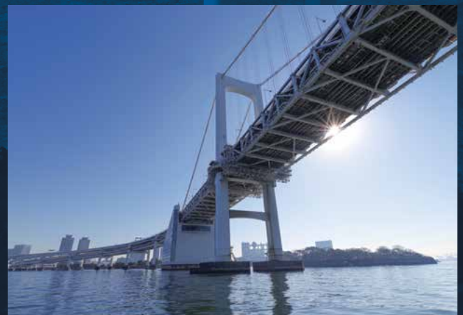
The Rainbow Bridge is designed with width considerations to accommodate the passage of large cruise ships.
