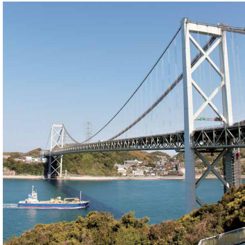
The Kanmon Bridge has a suspension structure that ensures a clear navigational channel for vessels passing through the Kanmon Strait.
